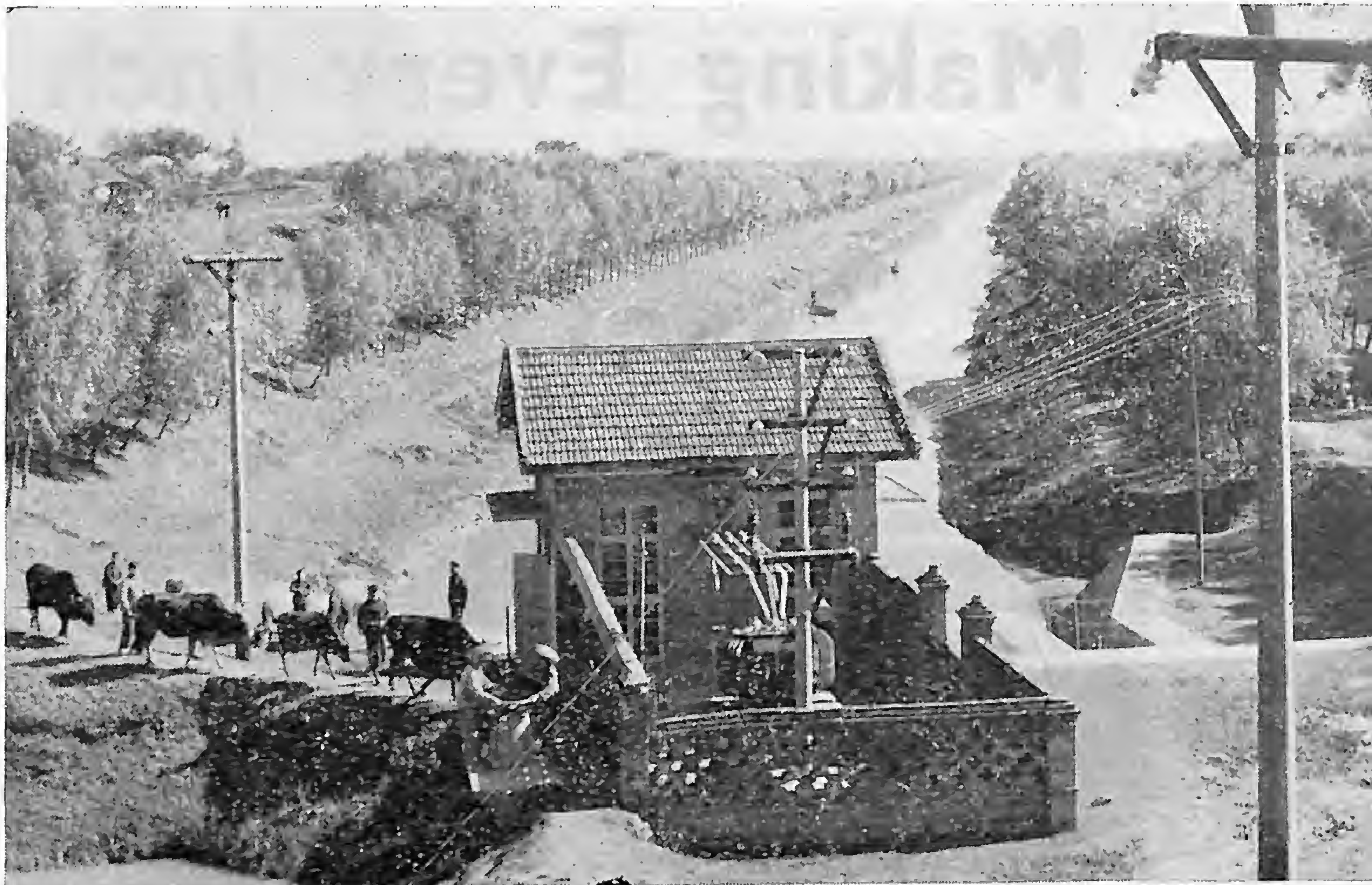
Today, instead of constant collapses of the dyke and crop failures, there are criss-crossing water channels, rows of willow trees, strong dykes and an electric pumping station. The low-lying waterlogged land has been turned into a granary.
